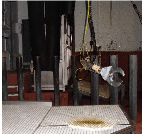
Hock cutter - 1 st stop post stabbing and suspension. Stun box can be seen behind.
